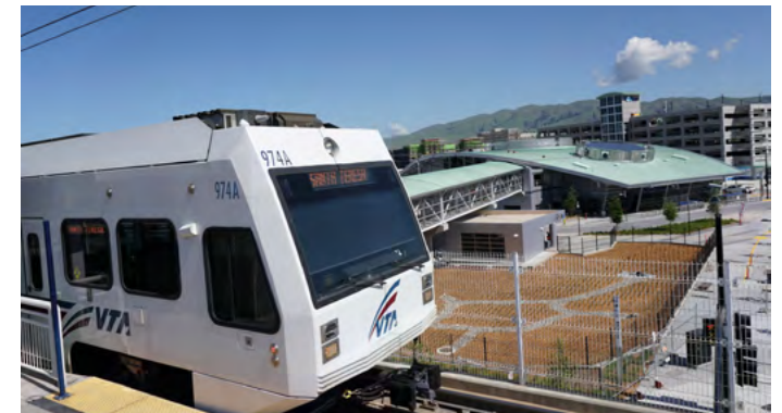
The new Milpitas BART station, in the background, connects to existing light rail service at the Great Mall Transit Center. [photo courtesy of the VTA]
