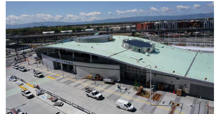
The Milpitas station was designed with extended curbs for employee shuttle buses and ride-share vehicles. [photo courtesy of the VTA]
